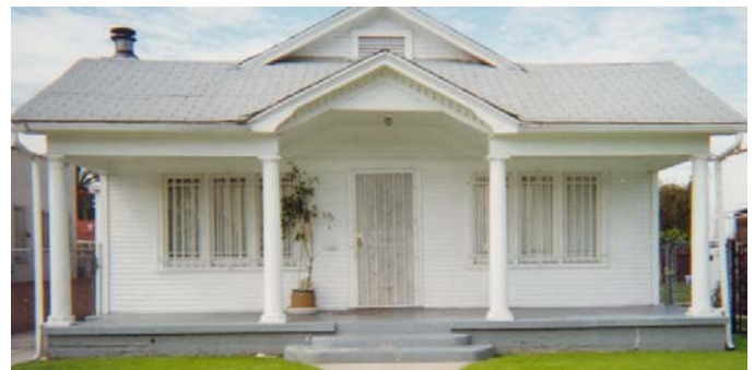
Fig. 1. Typical Single-Story House in the Northridge Earthquake Epicentral Area
